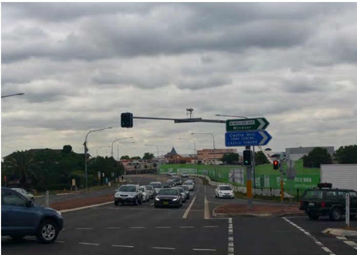
6 Site for the Castle Hill Train Station, currently under construction.
